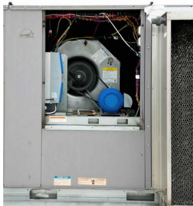
On the Los Cerritos Center rooftop, Motus Power retrofitted four RTU supply fan motors with Turntide Smart Motors and completed a stringent measurement and verification (M&V) process to obtain accurate baseline and post-installation readings.
